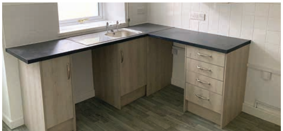
Finished kitchen units on external and party walls ©Peter Draper
