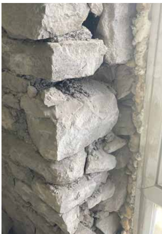
Reveals exposed prior to repair and IWI
